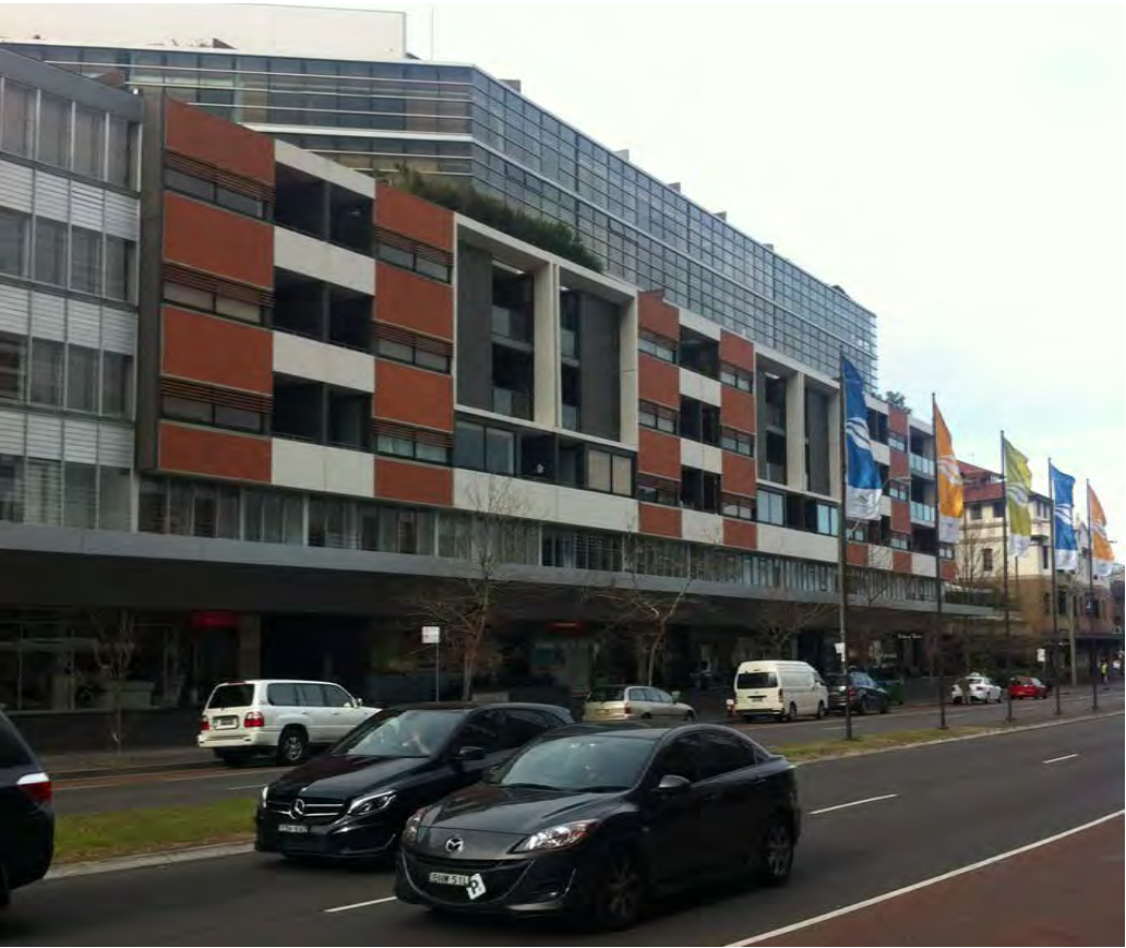
Anzac Parade 'Capella' with 5 storey built form to street edge and set back upper levels.
