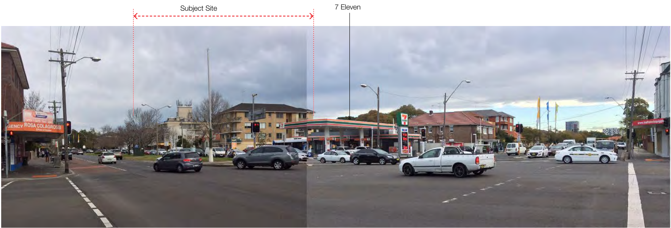
Corner of Todman Avenue and Anzac Parade - Looking south to subject site.
